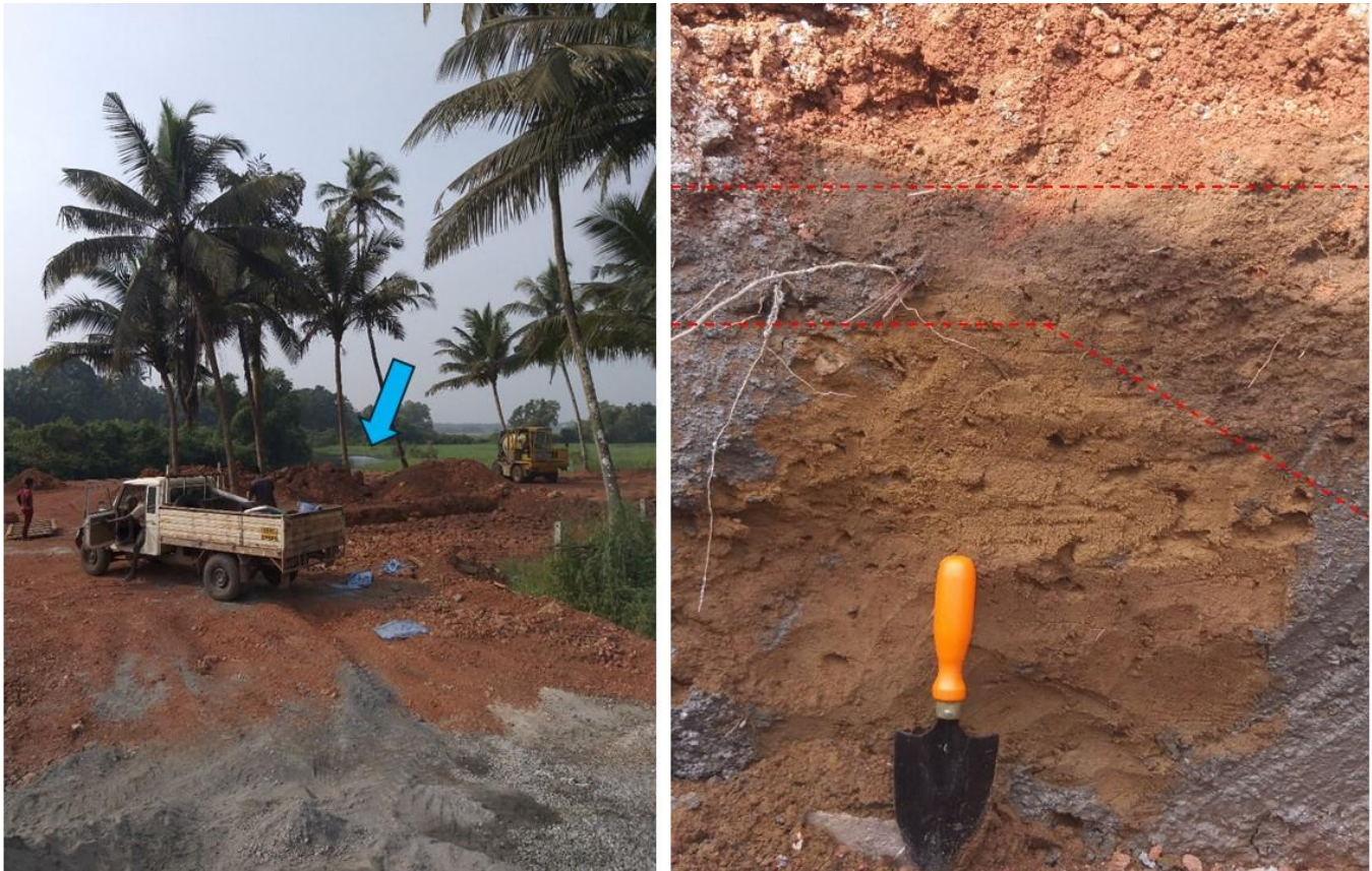
Figure 9. GO-2 sample, Construction site at the left with blue arrow denoting the tributary river location, to the right we can distinguish in a first visual examination three horizons in this alluvial soil type.
