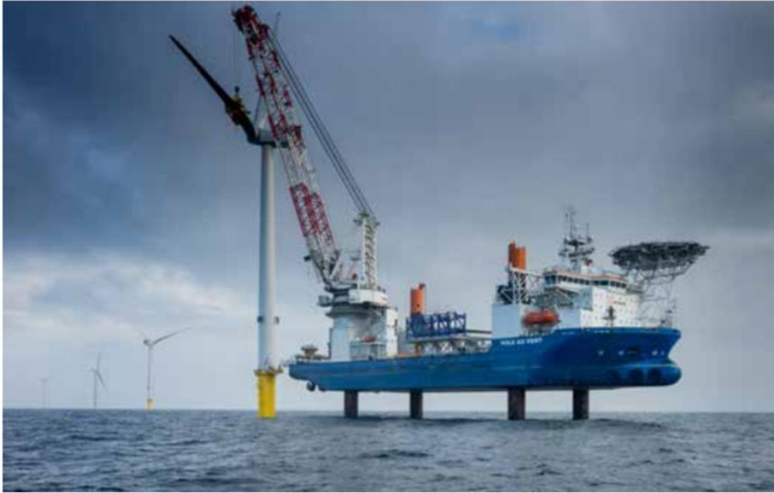
Figure 6.16 A jack up SIV vessel installing Dogger Bank wind turbines [96].
