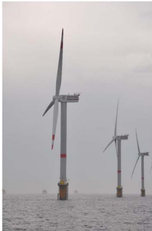
Figure 3.8 Large diameter monopile offshore wind turbines [45].
