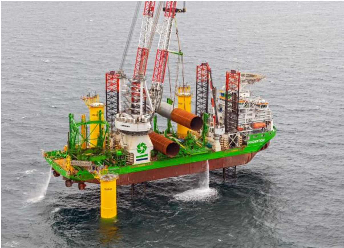
Figure 6.14 Installing Dogger Bank project's foundations by a jack up SPIV [75].
