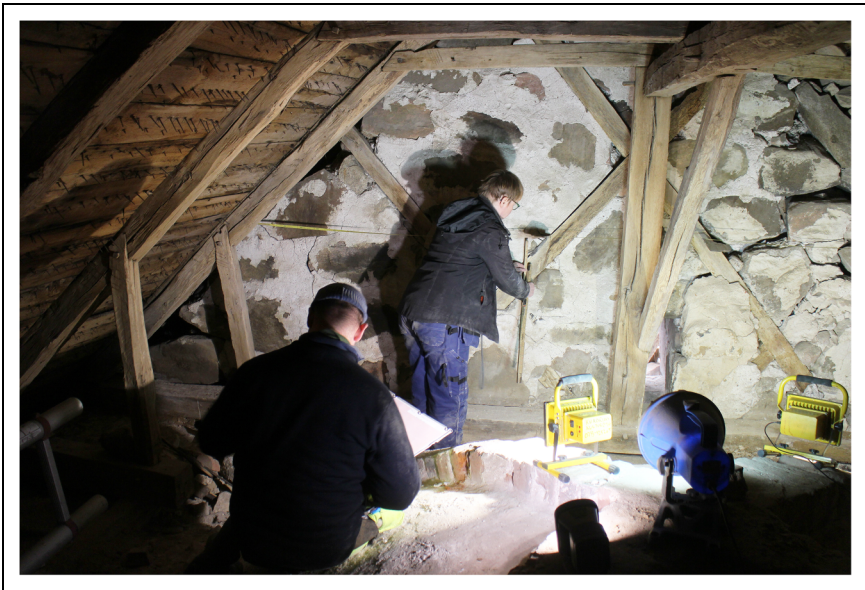
Figure 6. Documentation of 12th century roof truss embedded in the chancels gable and archaeological cleaning of Tåstarp church in collaboration with the archeologists from the museum Kulturen in Lund. Photo by the authors.
