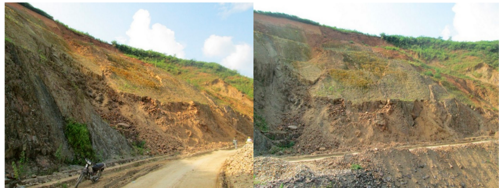
Figure 2. Two photos of the landslide on the slope wall of National Road 279, near the right bank of Nam Kim stream, Na Pa village, Muong Kim commune, Than Uyen district. Source: Vietnam Institute of Geosciences and Mineral Resources.
