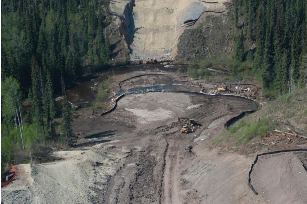
Figure 2: Ts'ellkay Kwa cleared for construction (Simmons, 2023c)
