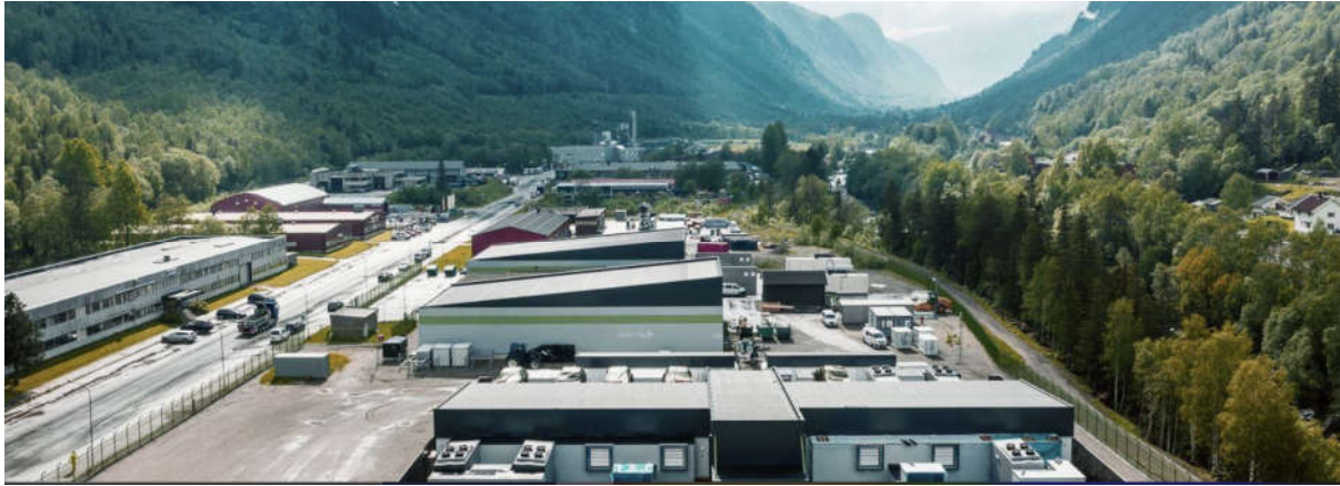
Figure 3.2: Data center of Telemark of Norway [35]
