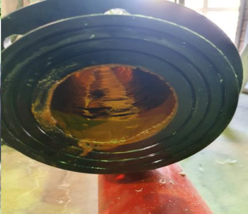
Internal view of the pipe straight section after the bend
