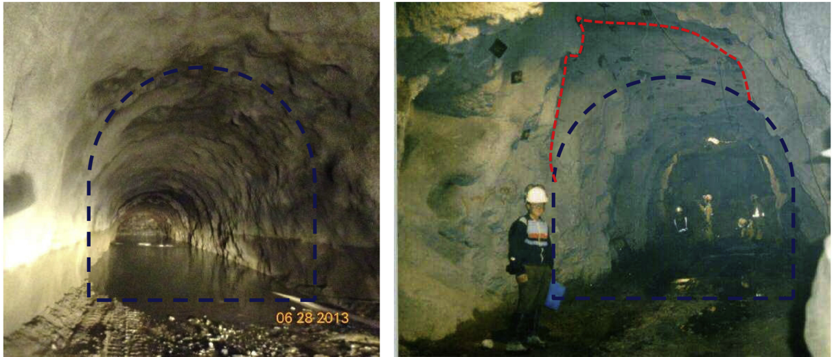
a. Relatively good quality tunnel contour (Upper Tamakoshi Project, Nepal)
