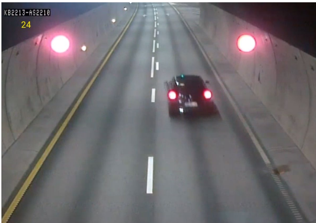
Figure 3-7 Warning of other drivers by lowering the speed limit and igniting emergency evacuation lights
