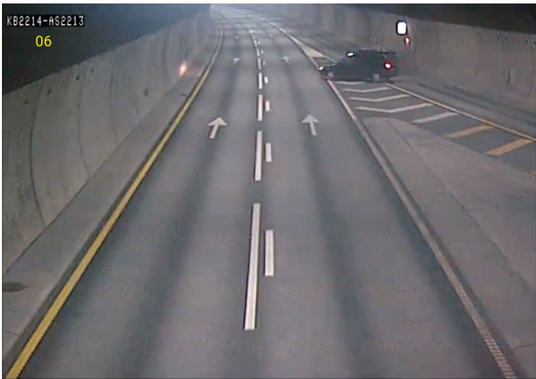
Figure 3-2 Car about to pass the road marking
