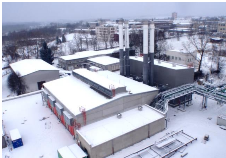
Figure 3-1: C-Energy power plant
