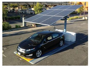
Figure 2.1: Stand-alone solar energy EV charging station [20].
