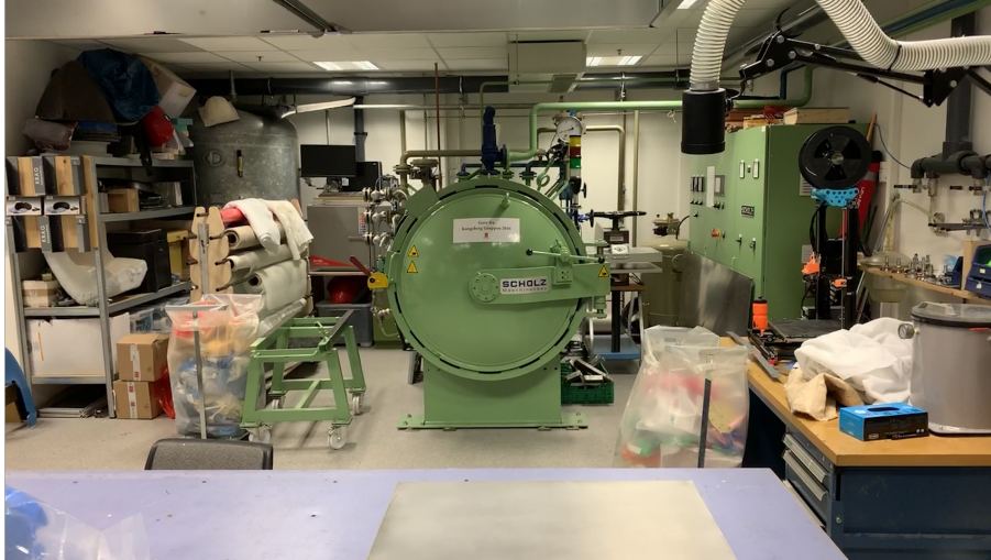
Figure 101: Autoclave at Krag Technology Lab
