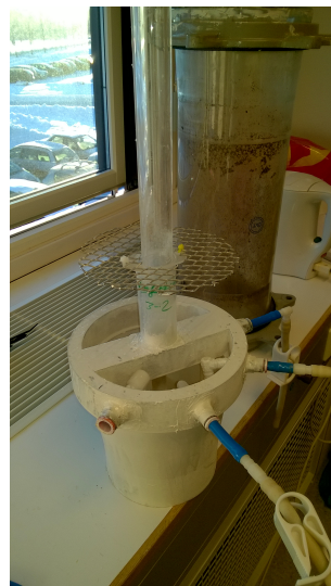
Figure 3–3: Three phase separator installed in pilot scale HyVAB ® bioreactor at NSO
