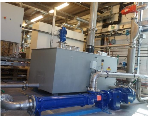
Figure 2B- 2. Pump and Tank section
