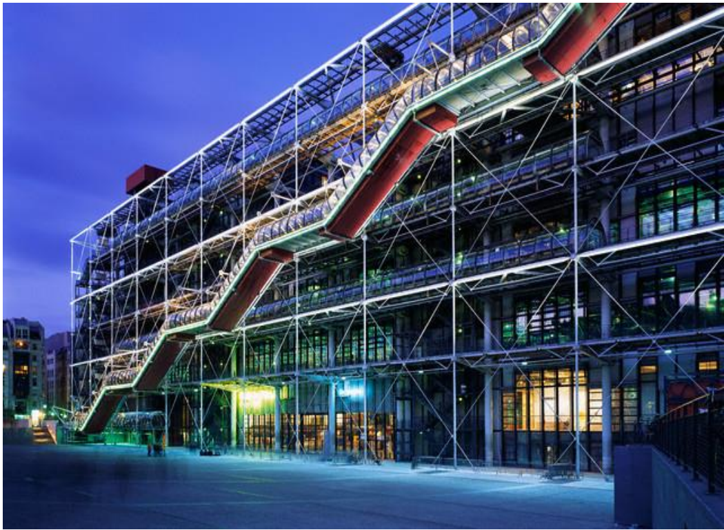
Figure 40. Georges Pompidou Centre, Paris. France, 1977, Renzo Piano, Richard Rogers. Main facade
