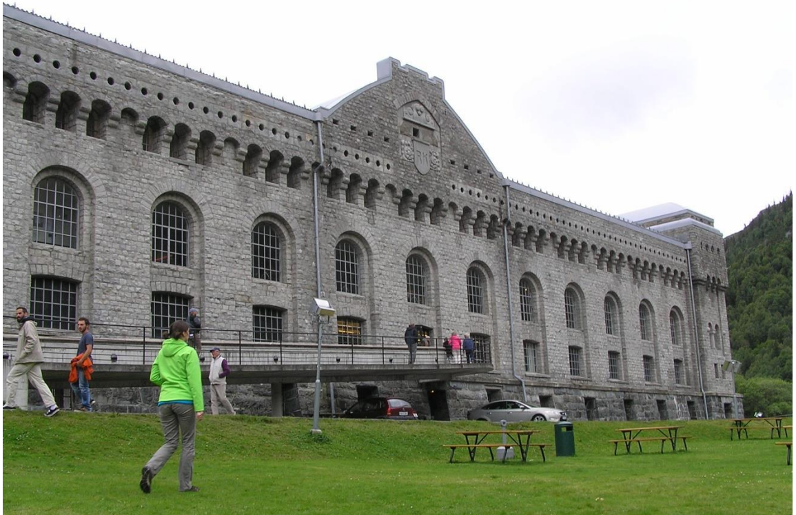
Figure 23. Vemork power station, Rjukan, Norway, 1911. Olaf Nordhagen
