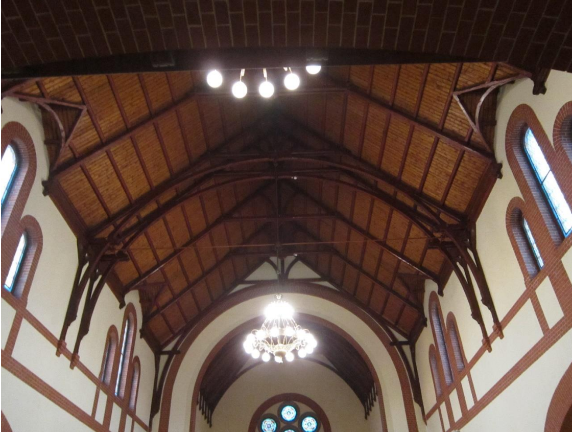
Figure 22. St. Johannes Church, Stavanger, Norway. 1907-1909, Jacob Sparre. Roof Construction
