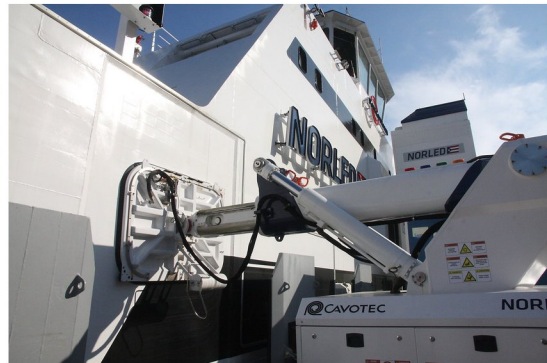
Figure 4: The vacuum based mooring system on “Ampere” (Stensvold, 2015c)
