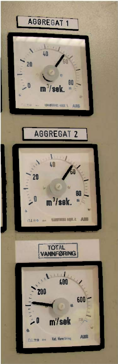
Figure 3-7: Flow rate for power production units.
