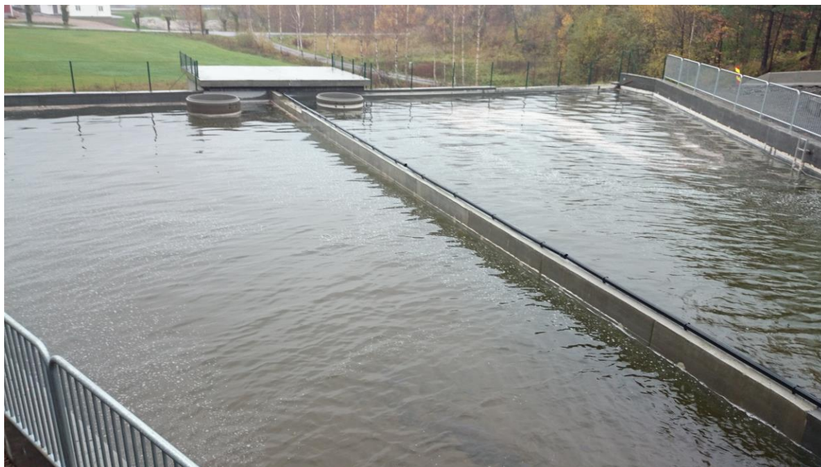
Figure 3. The two basins holding water after NaOH input in the treatment plant.
