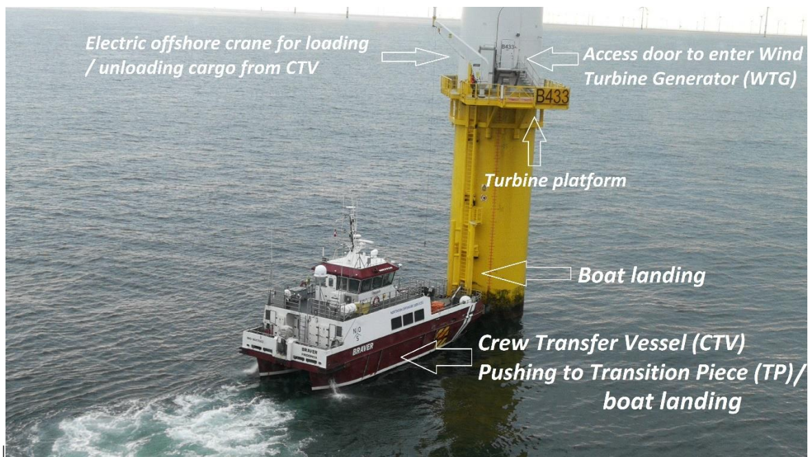
Figure 1 CTV pushing onto the boat landing in Borssele wind farm in the Netherlands
