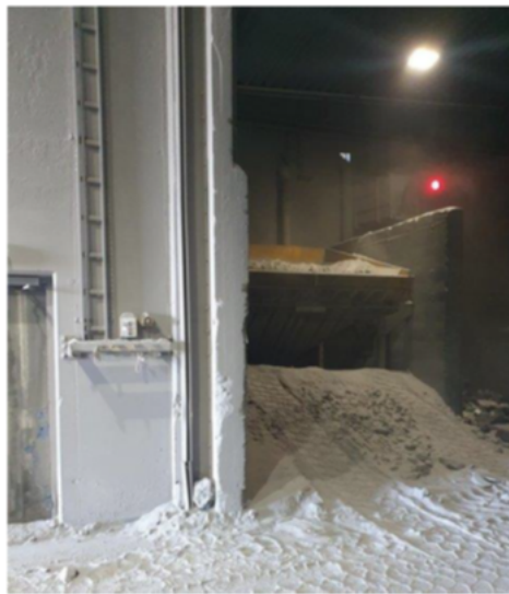
Figure 3.1 Hydro's storage area of ACM plant
