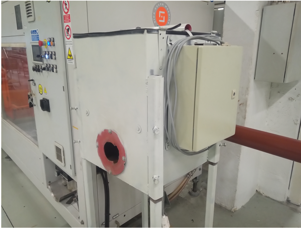
Figure 1.2: The proof-of-concept used to test the feasibility of inspecting
