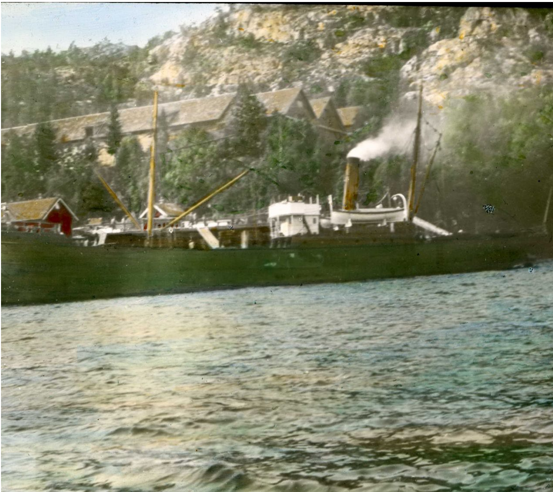
Figure 7.1. Steamship, possibly the Krystal , loading ice at Wiborg's Frøvik (Snekkevik) ice plant, probably 1900-1910. Hand-colored image, photographer A.B.Wilse, BKM.F.003112.
