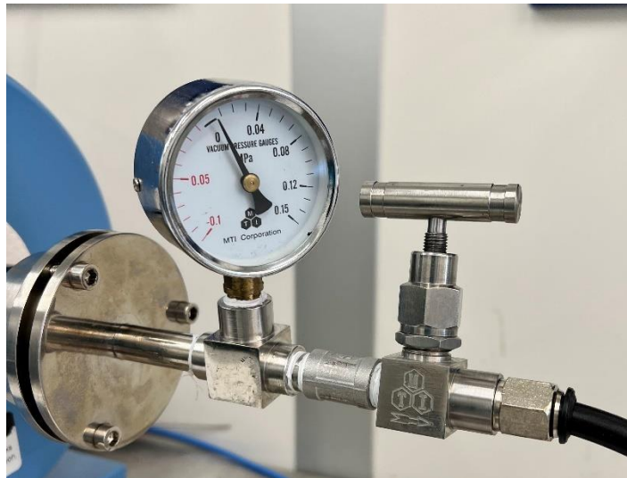
Fig 2-11 Atmospheric pressure indicating in pressure gauge of the tube furnace
