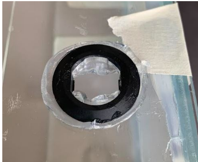
Figur 51: Sensor plugg montering.
