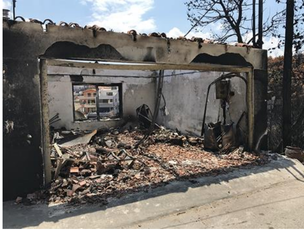
Fig. 1. Greatly damaged semi-confined space in the Mati fire (Greece, 2018) [4]
