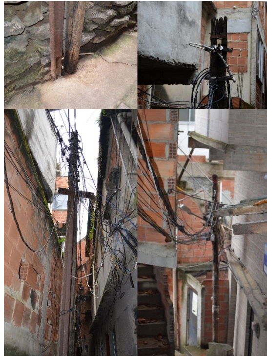
Figure 6: Public investments and resident solutions. This is a power supply from old railway sleepers that is still used today (Marcia, 2018).
