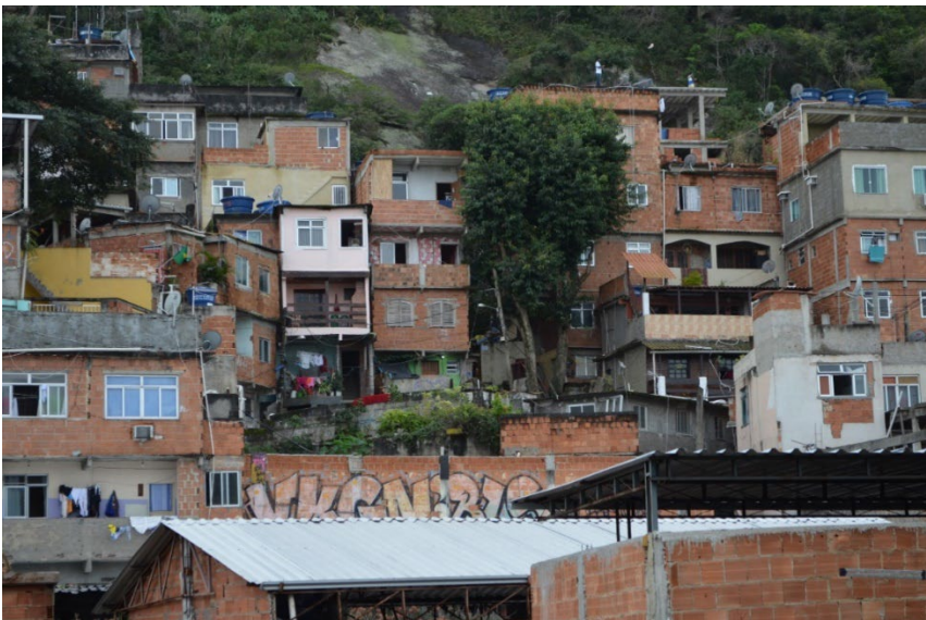
Figure 21 A photo of favela houses, illustrating the constructions that have taken place over the past decade. Many of the houses had expanded to four or five stories (photo by Marcia, 2018).
