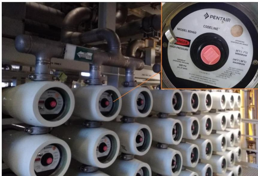
Figure 2.8: Feed side of a selection of membrane housings at Ivar Aasen SRU with nameplate indicating operating pressure and temperature.
