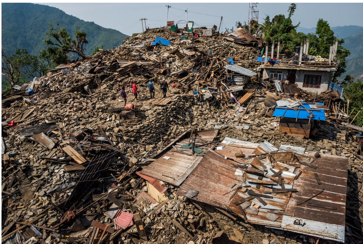
FIGURE 1.1: A glimpse of Nepal earthquake 2015. Picture Credit: Daniel Berehulak for New York's Time.
