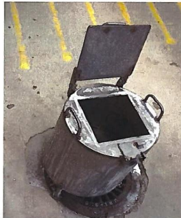
Figure 2: Container above drain, soft plug receiver
