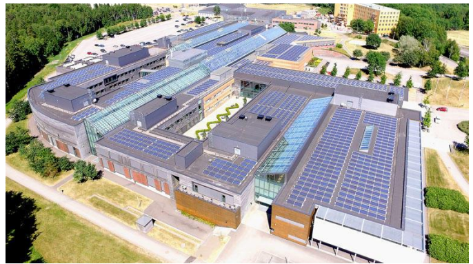
Fig. 1. PV system consisting of 1682 panels installed on USN rooftop.
