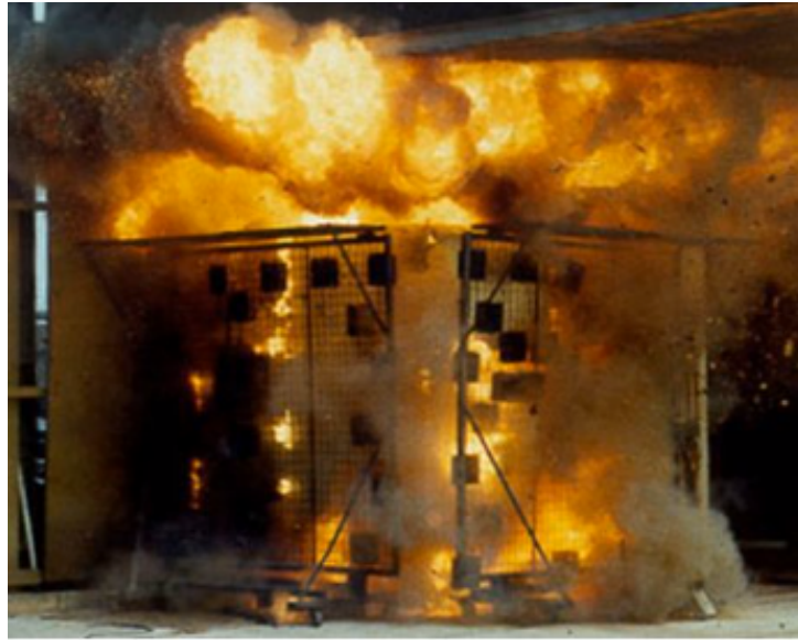
Figure 3.4: The potential consequence of an internal arc fault if the switchgear is not capable of handling the pressure and temperature increase [13]
