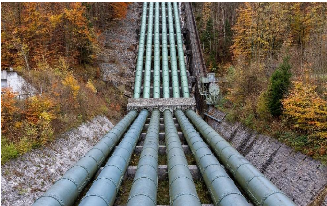
Figure 3.2: A multiple penstock arrangement [22].
