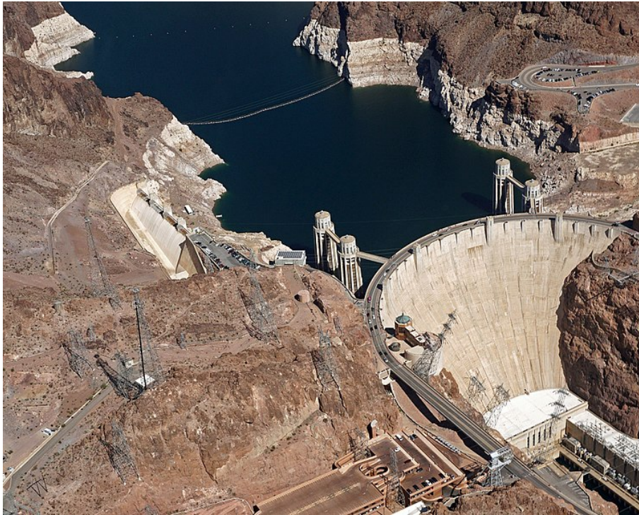
Figure 3.3: Aerial overview of the Hoover Dam [27]
