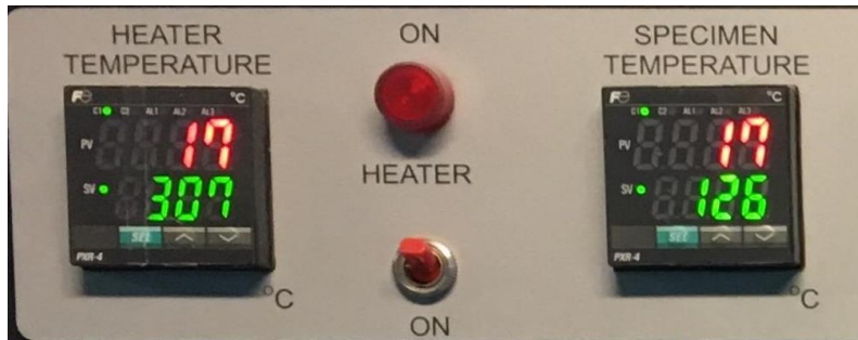
Figure 3.9: Digital display of PID controllers used for temperature control of the heater and the test specimen.
