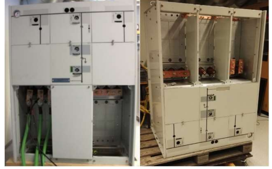
Fig. 6. Front view of the test object standing upright (left) and upside down (right).
