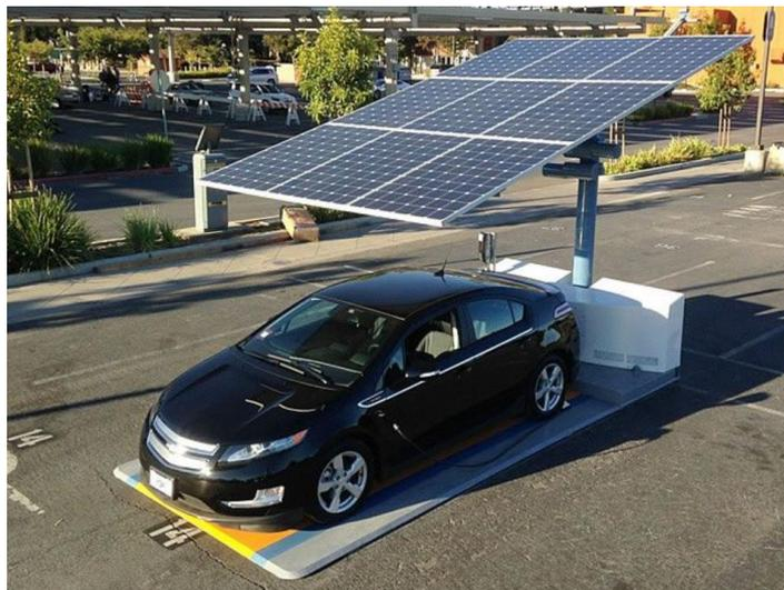
Figure 2.1: Stand-alone solar energy EV charging station [20].
