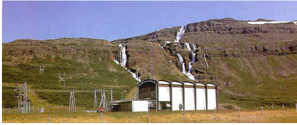
Figure 2. Power house of Mjólká 1 and Mjólká 2 (Westfjord Power Company 2018)
