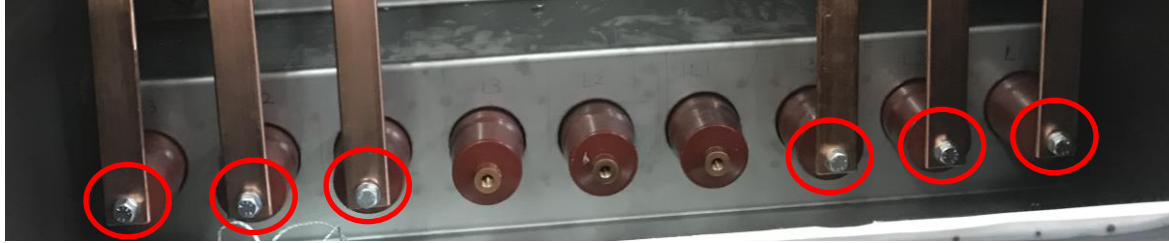
Figure 4.8 – Picture of which bolts and washers that are replaced during test 2
