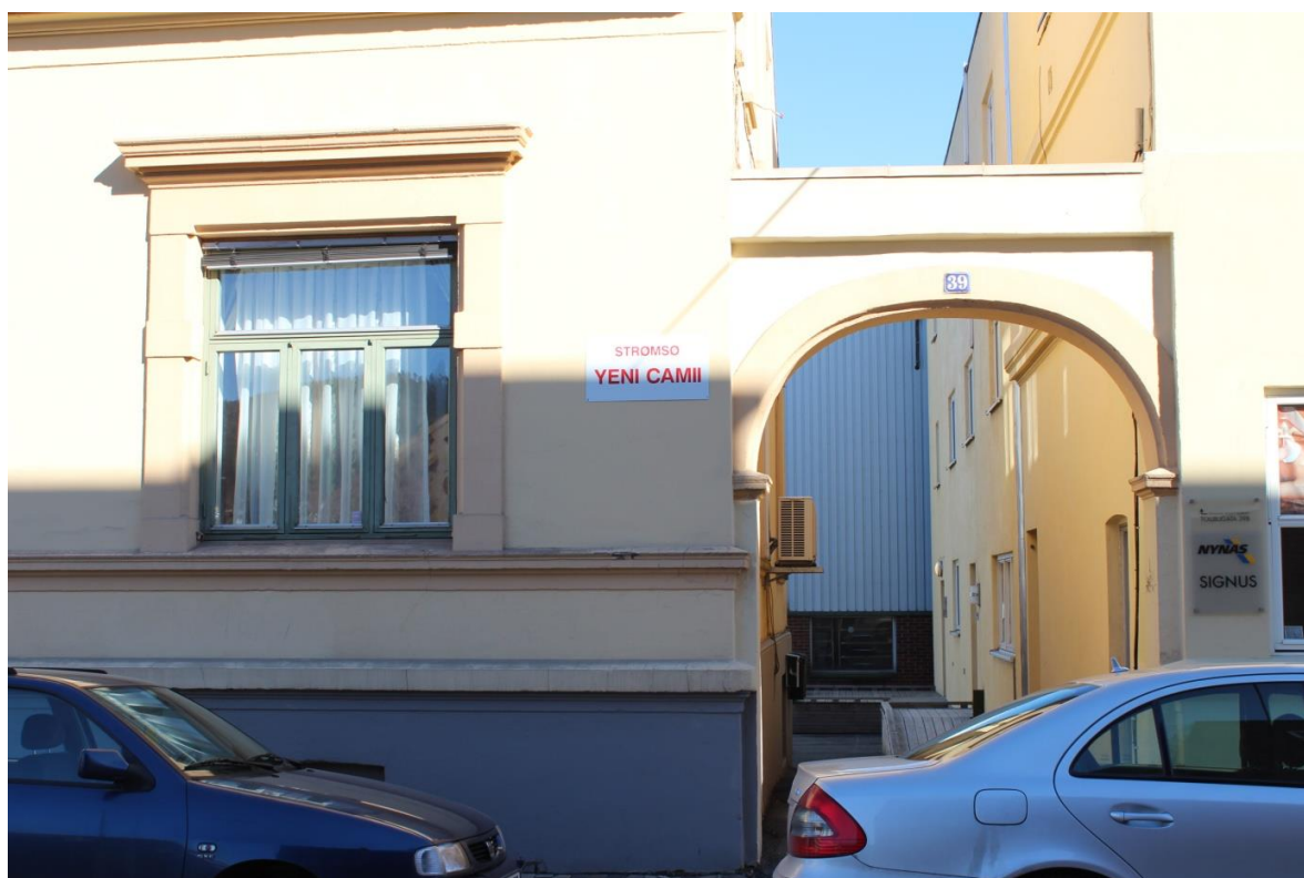
Photograph 19 Facade of a government Mosque in Strømsø district with an inscription in Turkish: 'Strømsø Yeni Camii' (Strømsø New Mosque).
