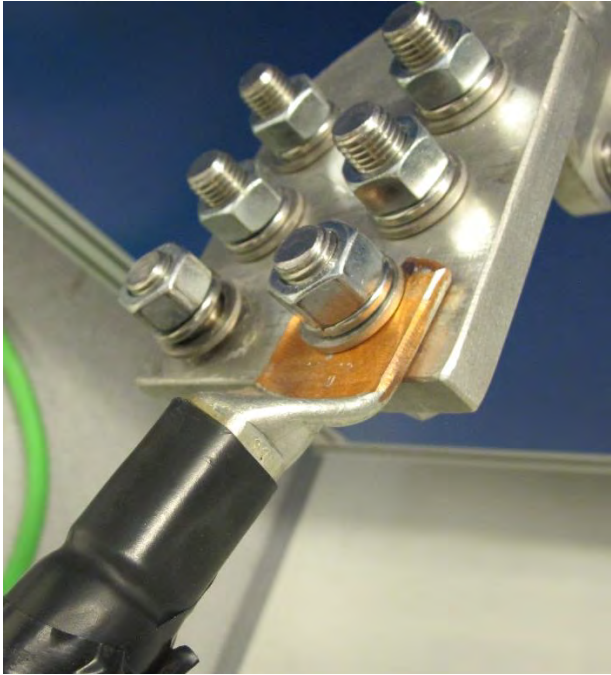
Figure 1 – how to connect cables
