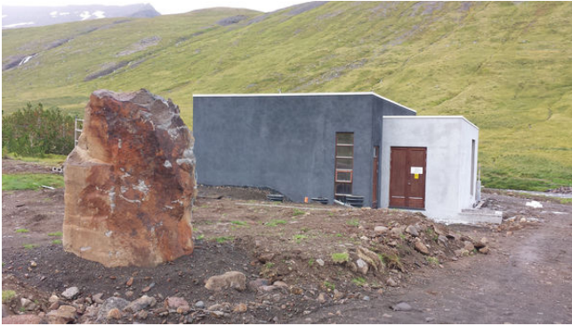
Figure 1. Power house of Fossárvirkjun ( Refurbishment of the Fossár hydro Power Plant 2015 )
