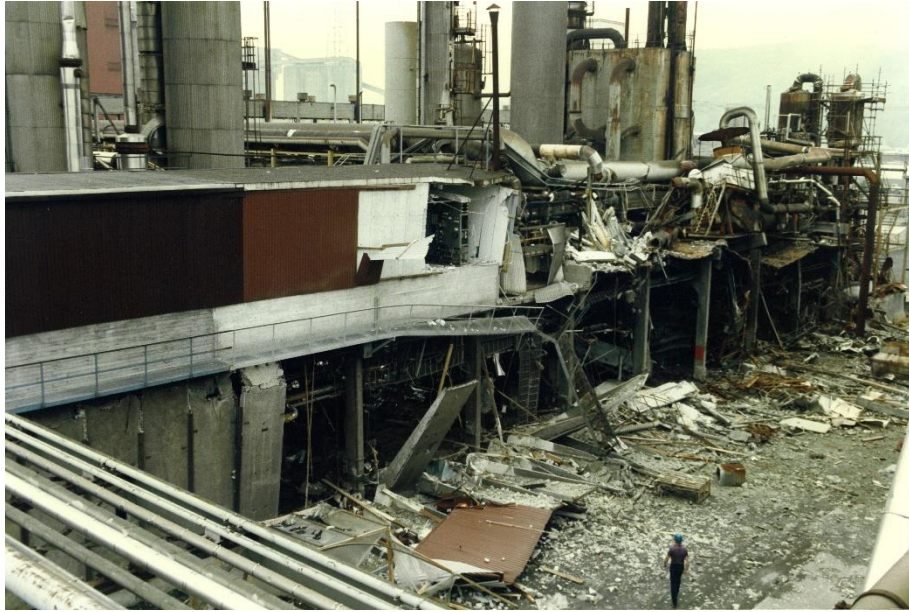
Figure 6.2 Photo of the northern wall of the factory building after the accidental explosion (Bjerketvedt and Mjaavatten, 1986). Photo: A. Kjellevoid.
