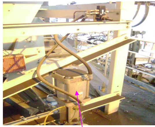
Figure 3.29: Shut down gate
