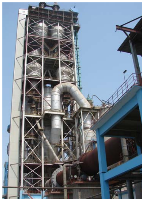
Figure 19: The kiln of Beijing cement plant with precalciner. (3 500 tpd)
