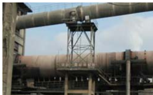
Figure 3: The first 2 000 tpd kiln with NSP in Jiangxi Cement Plant [8].
