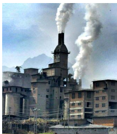
Figure 2: The shaft kiln [6].
