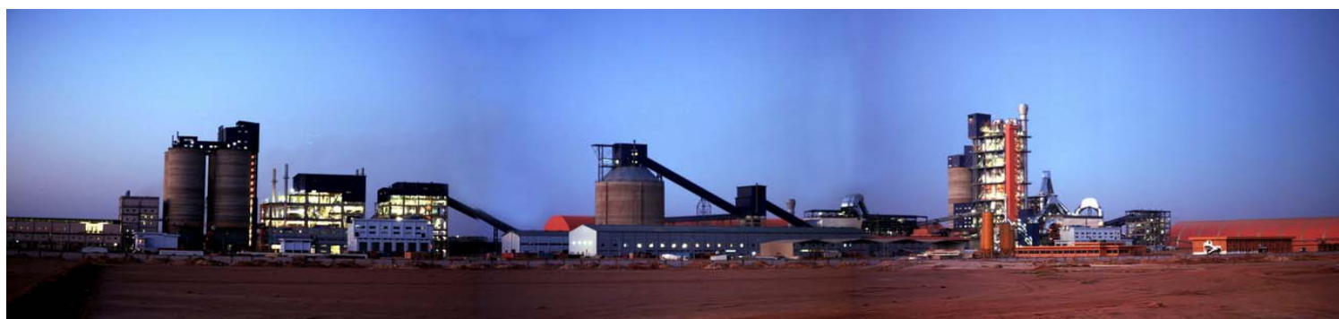
Figure8: 5 000 tpd cement production line in Saudi Arabia made by Sinoma [12].
