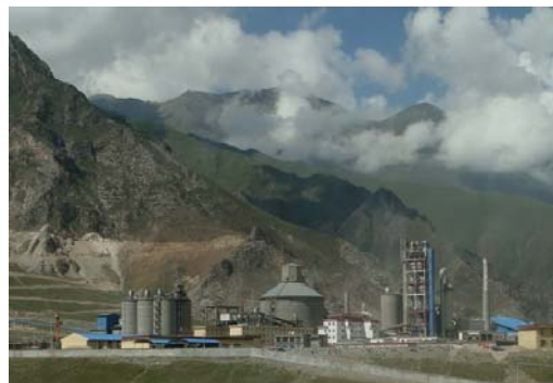
Figure9: Tibet Gaozheng cement plant with 3 730m [14].
