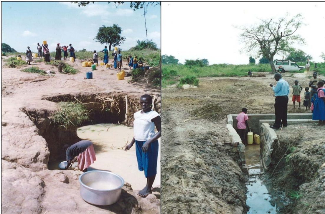
Figure 2: From unimproved (left) to improved (right) water source (Source: Author, 2005).
