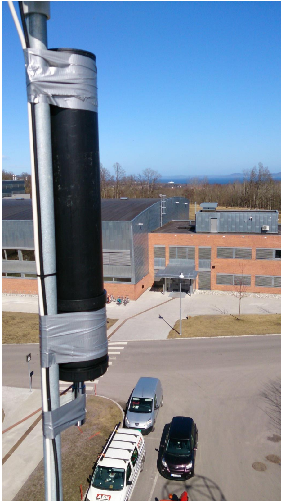
Figure 6b. Sensor 1 view. The sensor is weather protected inside a black plastic cylinder, taped to an existing mast on the roof of Vestfold University College. One of the Horten-Moss ferries is visible in the horizon.
