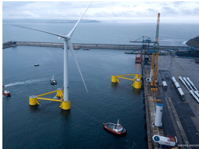
Figure 4. WindFloat semi-submersible assembly in port. Credit: DOCK90 (Power-technology, 2020)
