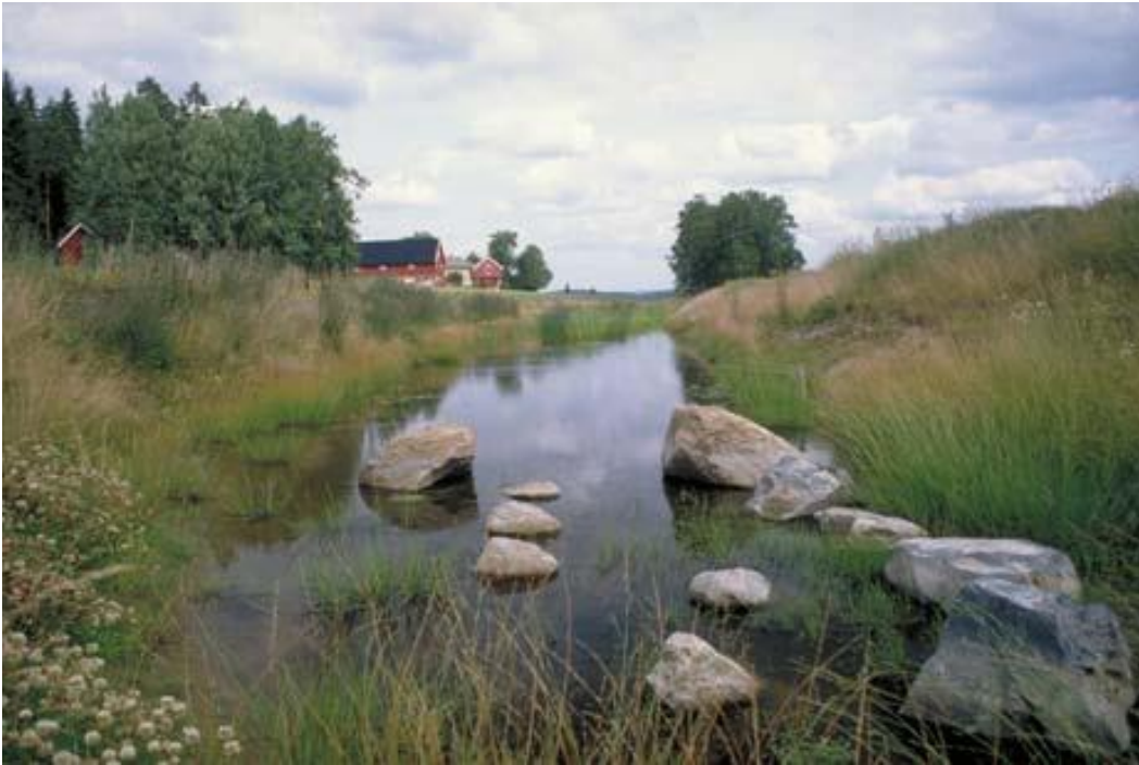
Figure 2-1 Overview of waterflow in stream through constructed dams
