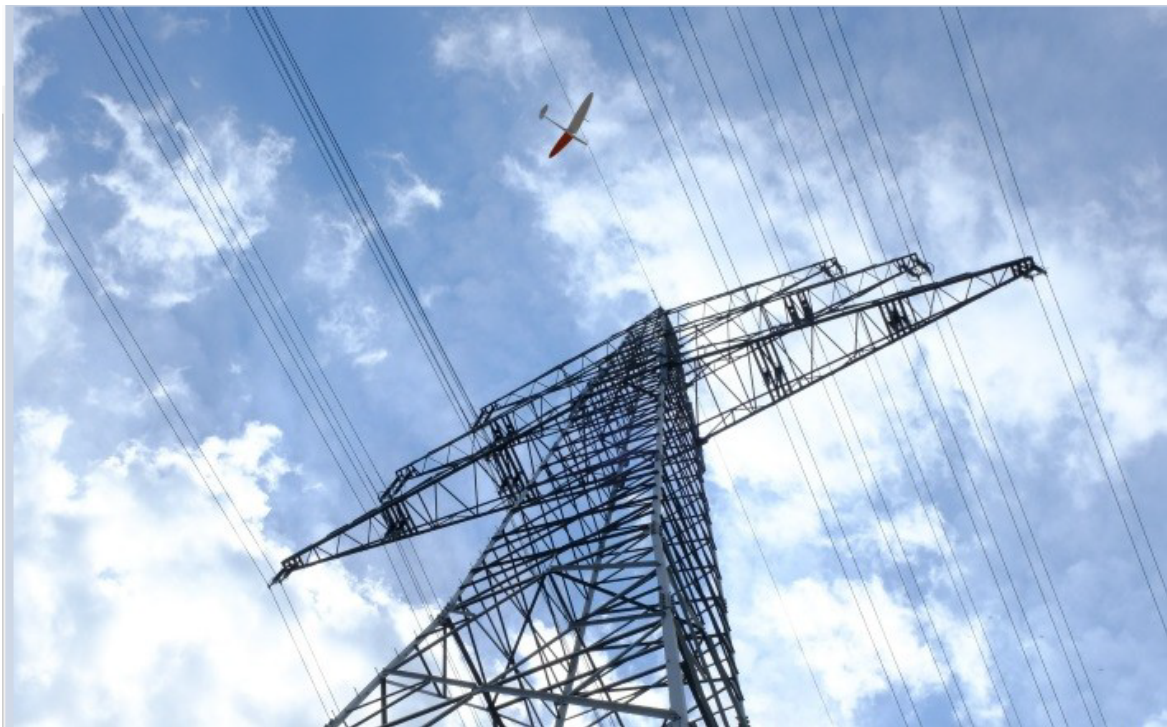
Figure 2.7: Power line inspection by using BVLOS, Delair Tech [21]
