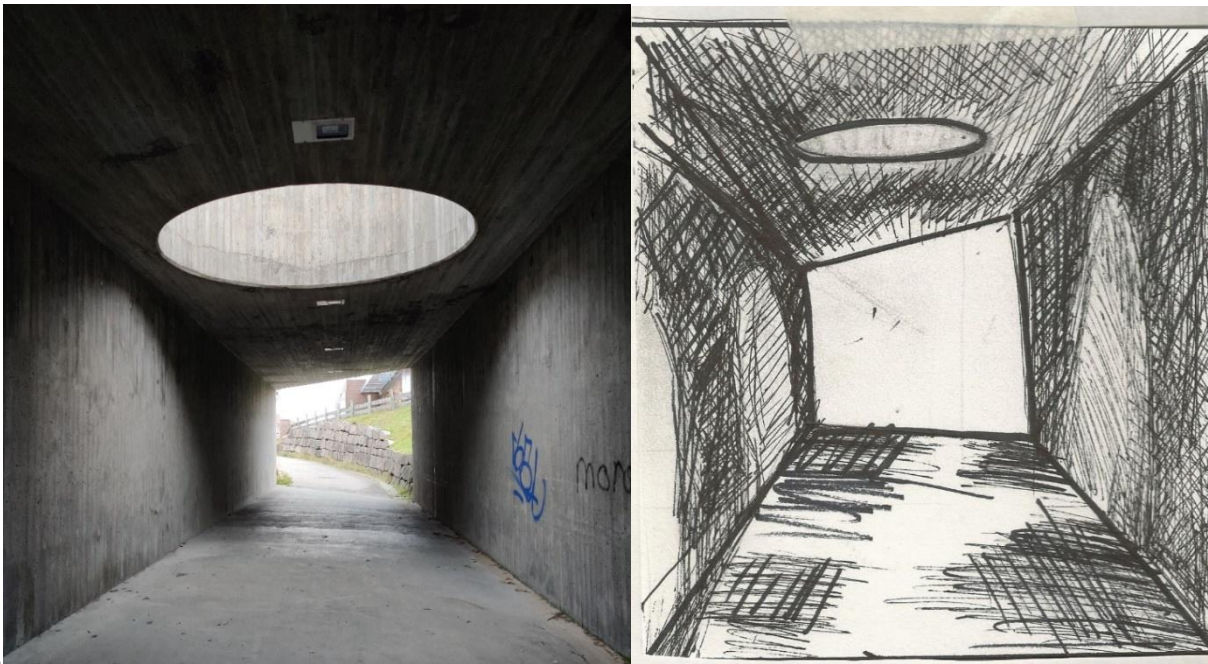
Picture 17 and 18: Top -Left: Interior view of Myren underpass in Skien. Right top: Underpass entrance view sketch (Private photos)
